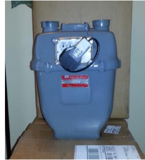
Figure 17. IMAC system pulser attached to the natural gas flow meter
